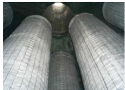
Wet Catalysis Candle Filters below vessel exit
